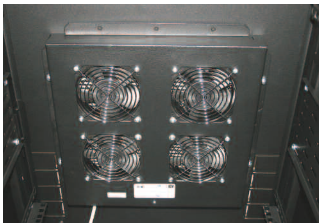
Image shows roof mounted Smart Net Fan Unit fitted in cabinet
