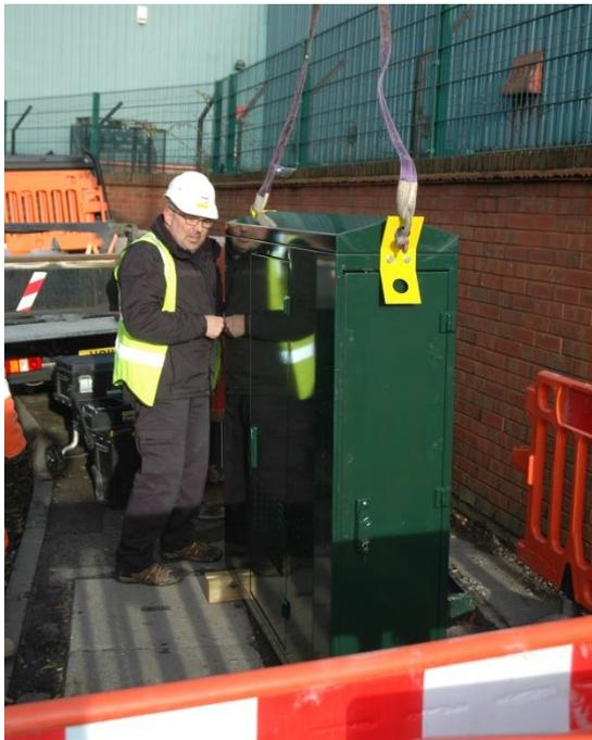
*Image #1 Caption: Example of outdoor enclosure with thermal management system and cable access via base ducting being installed by Cannon Technologies.*
