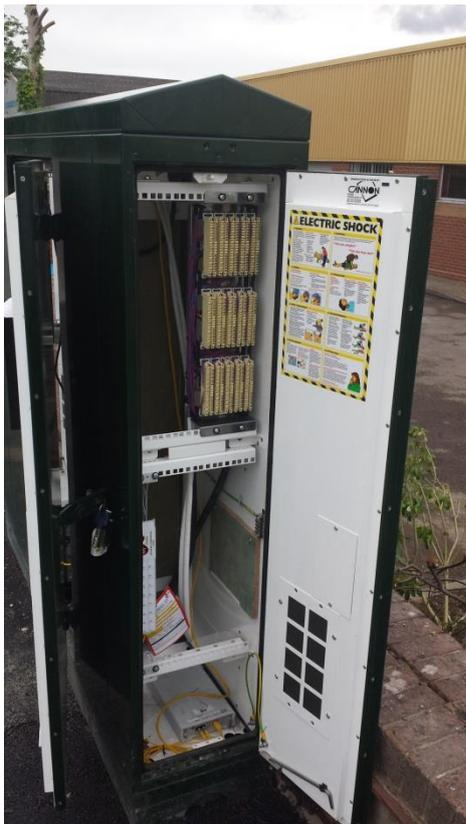
*Image #3 Caption: Example of vertical stack equipment compartment*
