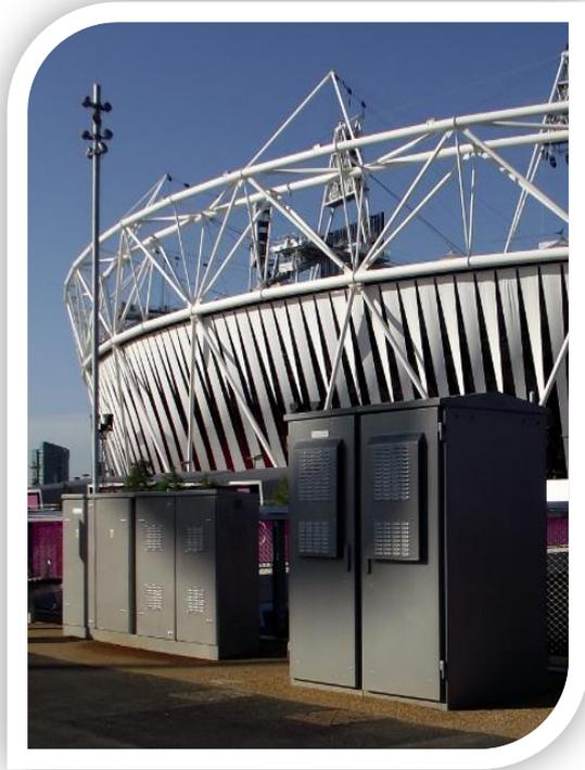
*Image #2 Caption: Enclosure installation at base of London Olympic Stadium providing security and thermal management to sensitive electronic CCTV equipment.*
