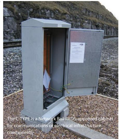
The C-TYPE is a Network Rail PADS-approved cabinet for communications or electrical infrastructure components
