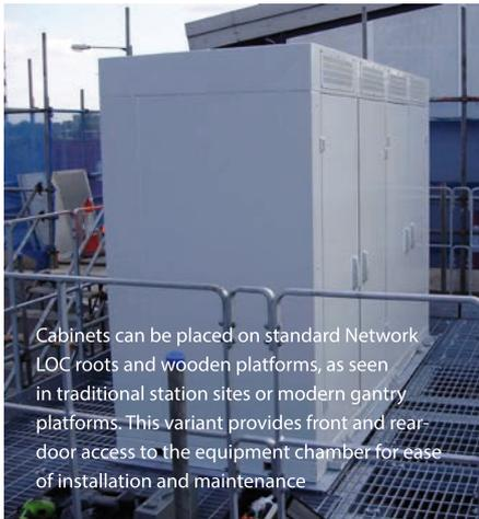
Cabinets can be placed on standard Network LOC roots and wooden platforms, as seen in traditional station sites or modern gantry platforms. This variant provides front and rear-door access to the equipment chamber for ease of installation and maintenance
